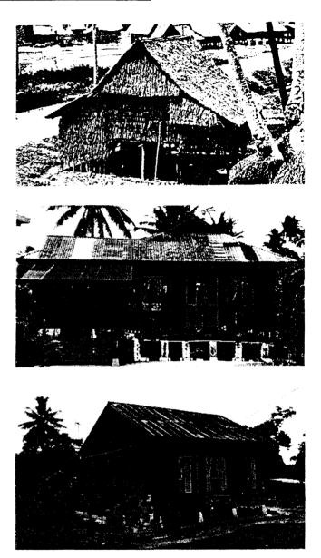
Fig. 1. *Top*, a 19th-century photograph showing a *kampung* house completely walled and roofed with *atap* thatch (Courtesy National Archives of Singapore); *middle* and *bottom*, examples of 20th-century *kampung* houses roofed with zinc sheet, a material which allows shallower and more rationalized forms of roof construction. (Photos: Ho-Yin Lee)
