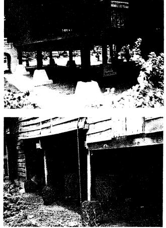
Fig. 3. House-posts of *kampung* houses resting on plinths of cast concrete (*top*) and blocks of natural stone, probably laterite (*bottom*). (Photos: Ho-Yin Lee)
