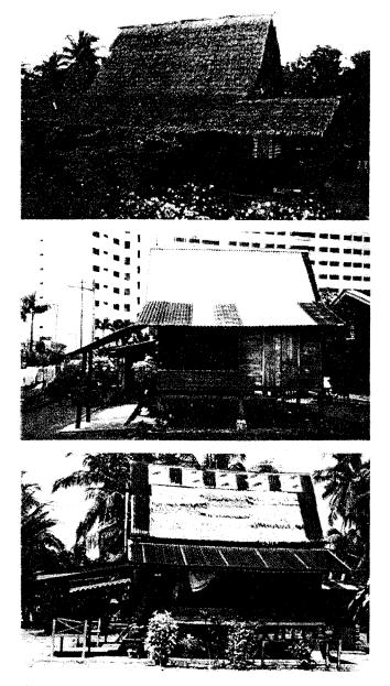
Fig. 2. Transformation of roofing method: from *atap* thatch (*top*), to zinc sheet (*middle*), to zinc-*atap* composite (*bottom*). (Photos: Ho-Yin Lee)
